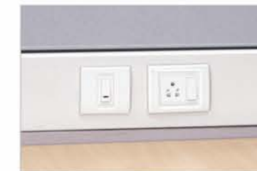
Switches mounted on Raceway
